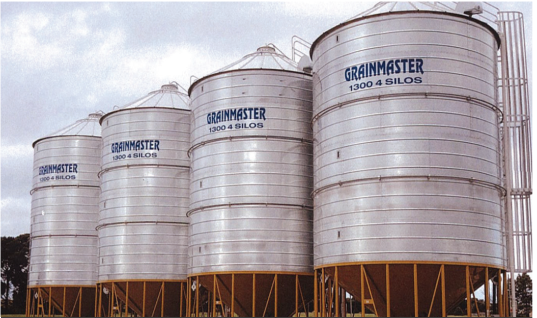
206t, $45,000 + concrete each. 90ft auger/tubulator to fill Supplier: SA Grain Services
