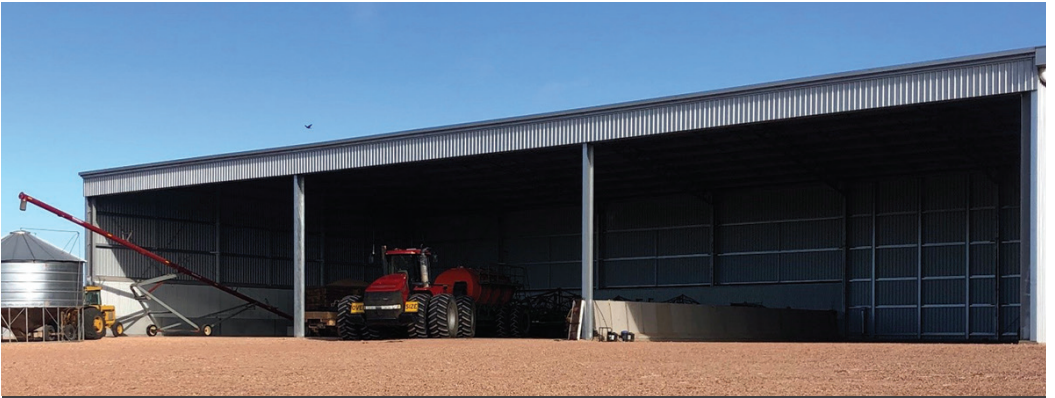
Redden Bros sheds 48.5m x 28m x 7.5m [Waddikee] $425,000 includes tank, pad, concrete [EP example 2019]
