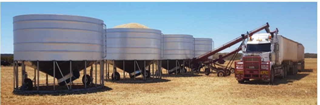
Welke silo DIY, approx. $9,000 for kit ex WA, plus $3,000 on farm labour $12,000 to complete. Can fit 11 DIY kits on a semi-trailer.
