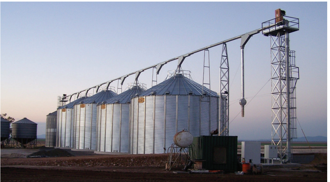
737t, $131,000 incl concrete 1331t, $156,000 each incl concrete, supplier: AGCO - GSI Silos Tim Pfeiffer
